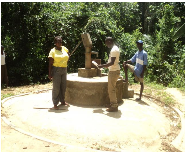
The newly constructed Hand pump at the Farm/Peace Village
